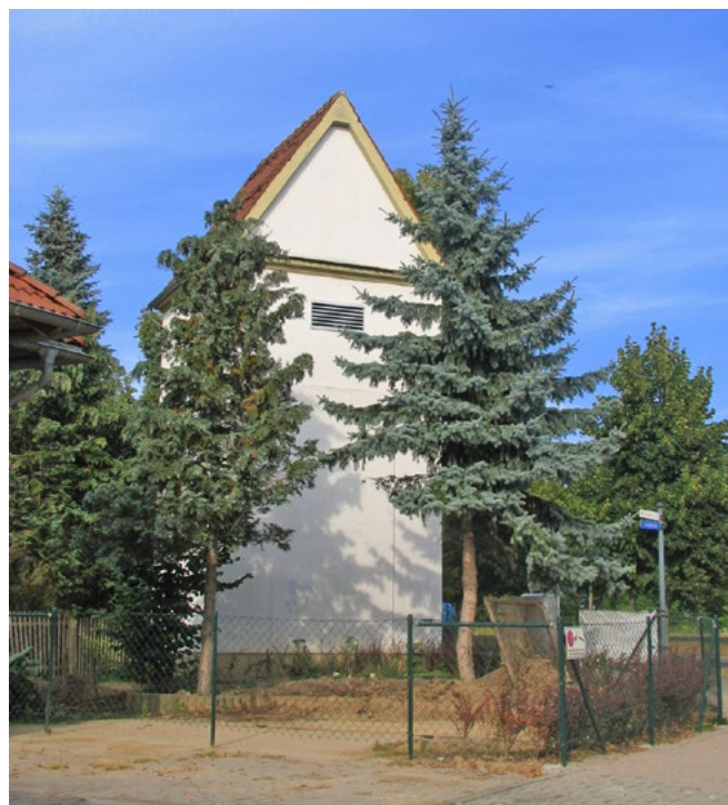
Turmstation in Kranichfeld, 2013
